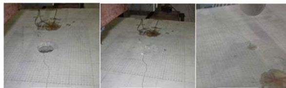
Figure 6. Damage incurred on impact side of the RC100 panel: A) after the first impact, B) after the second impact, C) after the third impact
